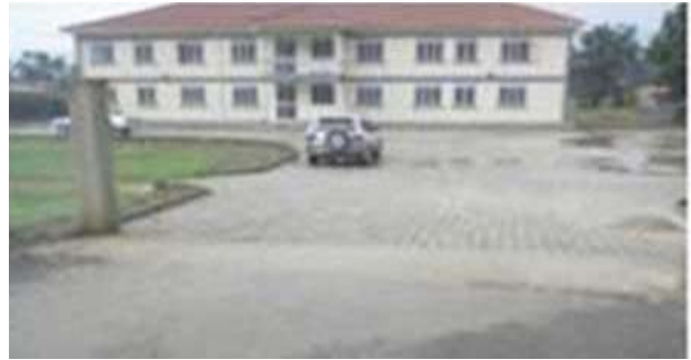
Completed Kabale Police station
