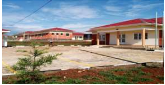
Completed Mitooma Justice Centres
