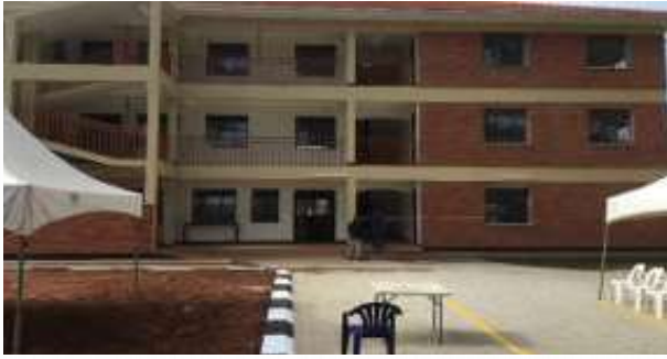
Completed Masindi High Court
