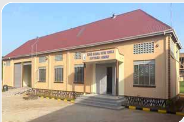
Regional Vehicle maintenance Centre in Gulu
