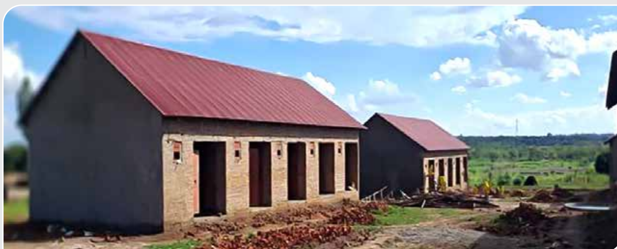
Staff houses on the finishing level at UG. Prison Nakasongola
