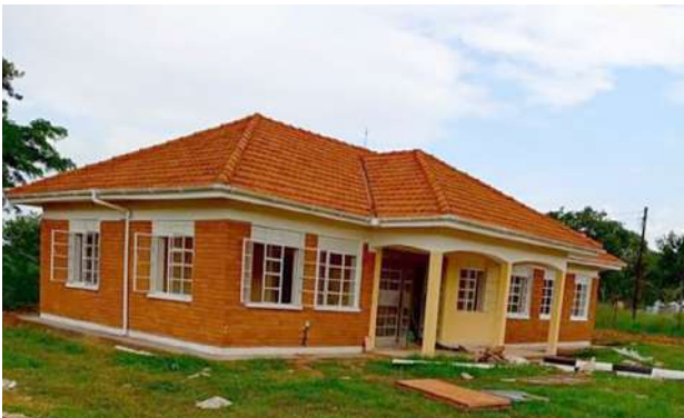
Renovated Abim RSA's Office showing newly fitted gutters, painted walls and windows, cleaned roof tiles
