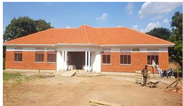
Construction of Soroti ODPP Regional Office
