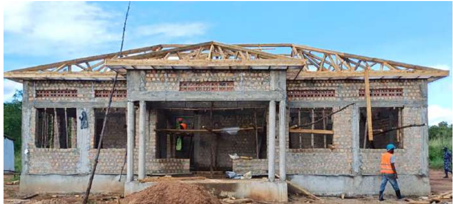
Construction of RSA’s office at Madi Okollo
