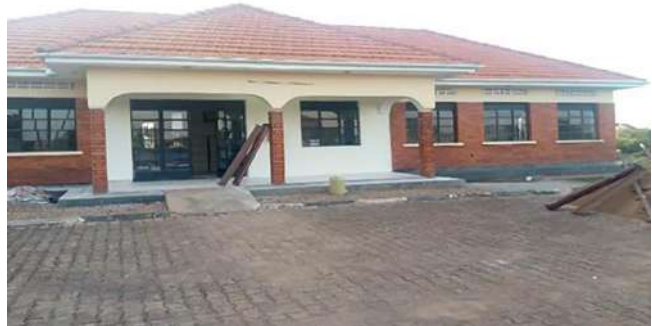
Renovation of RSA's office in Apac
