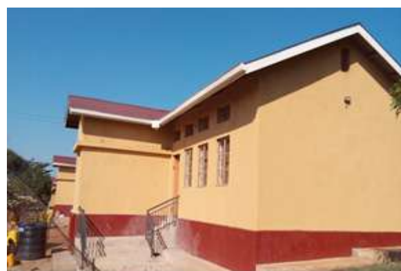
Completed renovation of Prisoners wards at Tororo
