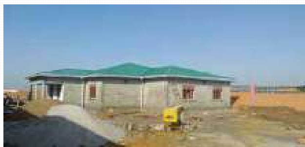
Detention facility for irregular immigrants near completion
