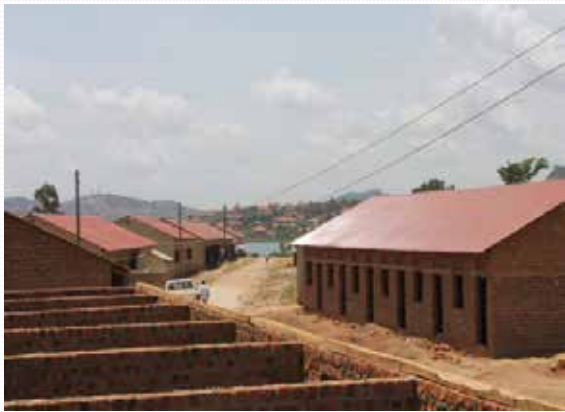
Construction of low cost staff houses at Luzira barracks
