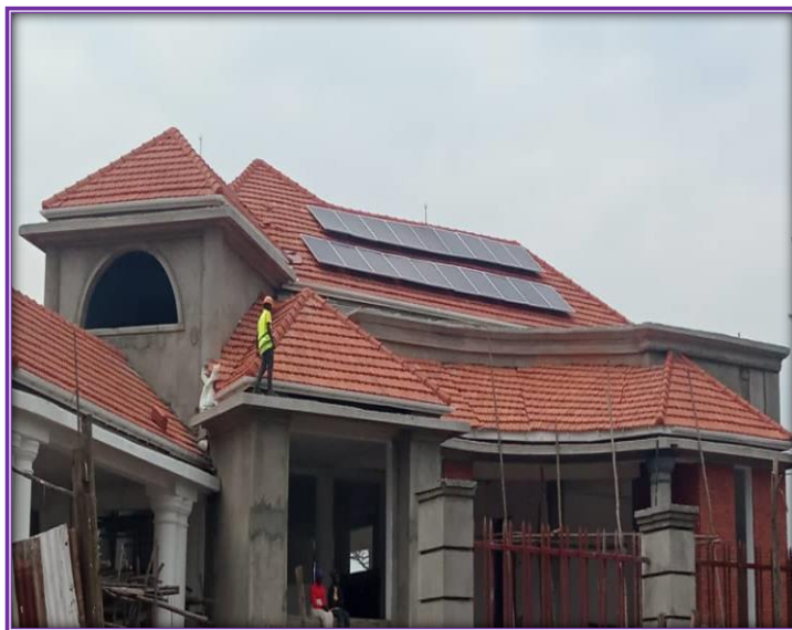
Construction of MoJCA Fort Portal Regional Office underway
