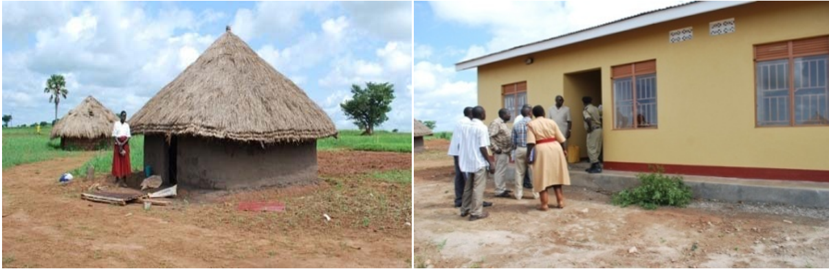
Oyam Prison Staff quarters before and after construction
