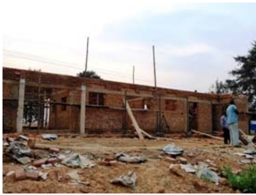
Kanungu Court Hall block under construction
