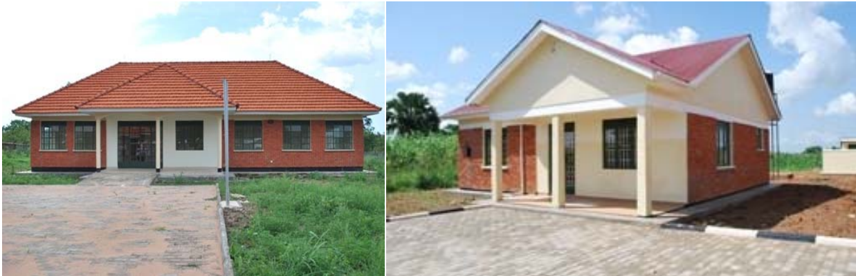
Adjumani DPP offices and Amolator Staff quarters
