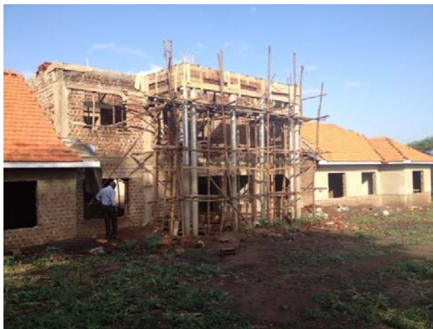
Mini JLOS building under construction in Moroto
