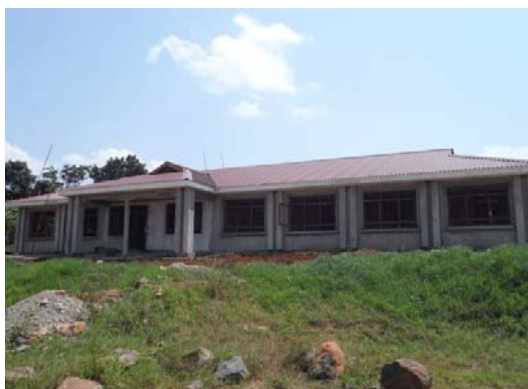
Mbarara Regional Laboratory at final stages of construction
