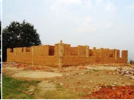
Kanungu Police Station under construction
