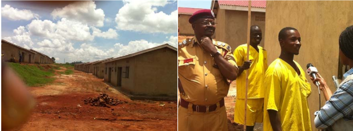
Low cost staff house built using prison labour at Luzira prison
