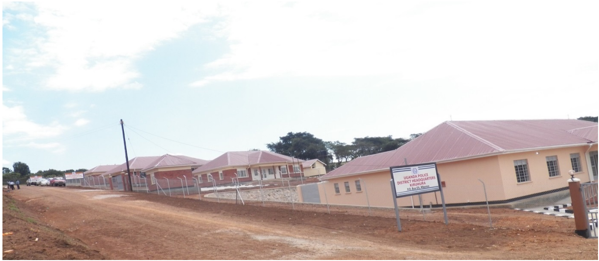
Figure 2 Kiruhura Justice Centre, a one stop centre for Policing, prosecution and Court services
