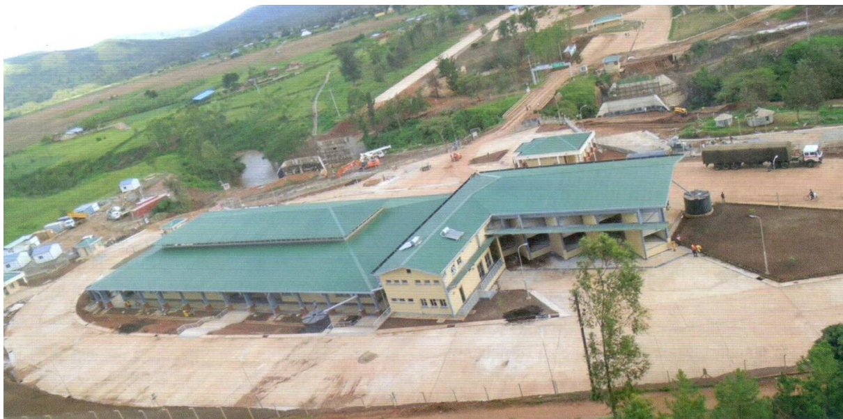
Figure 3 an aerial view of the Miram Hill one stop border post
