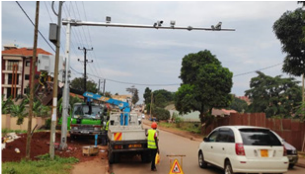
CCTV installation along roads within KMP and National Command center under construction at Naguru
