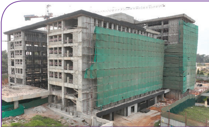
JLOS House 2 (Police Headquarters) under construction
